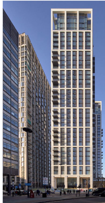
Fig. 33 Example of approach to the facade treatment of tall buildings. Southbank Place, London, Squire and Partners.
