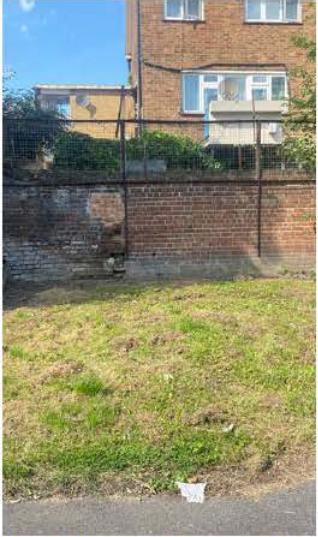
Viewpoint 01: Existing northern boundary wall adjacent to Penshurst Rd plots.
