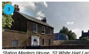
Station Masters House, 52 White Hart Lane
