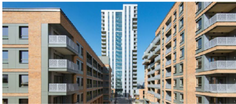
Fig.21 - Brook House Development
